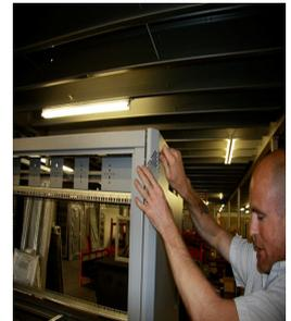
Insert roofing bolt through the top cover and then through aluminium spacer and screw into captive fixing in top of cabinet.
