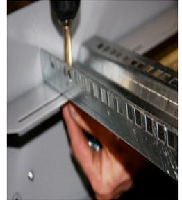
Attach vertical infill panels to the front right and left profiles only. NB these are only used on 800mm wide cabinets.
